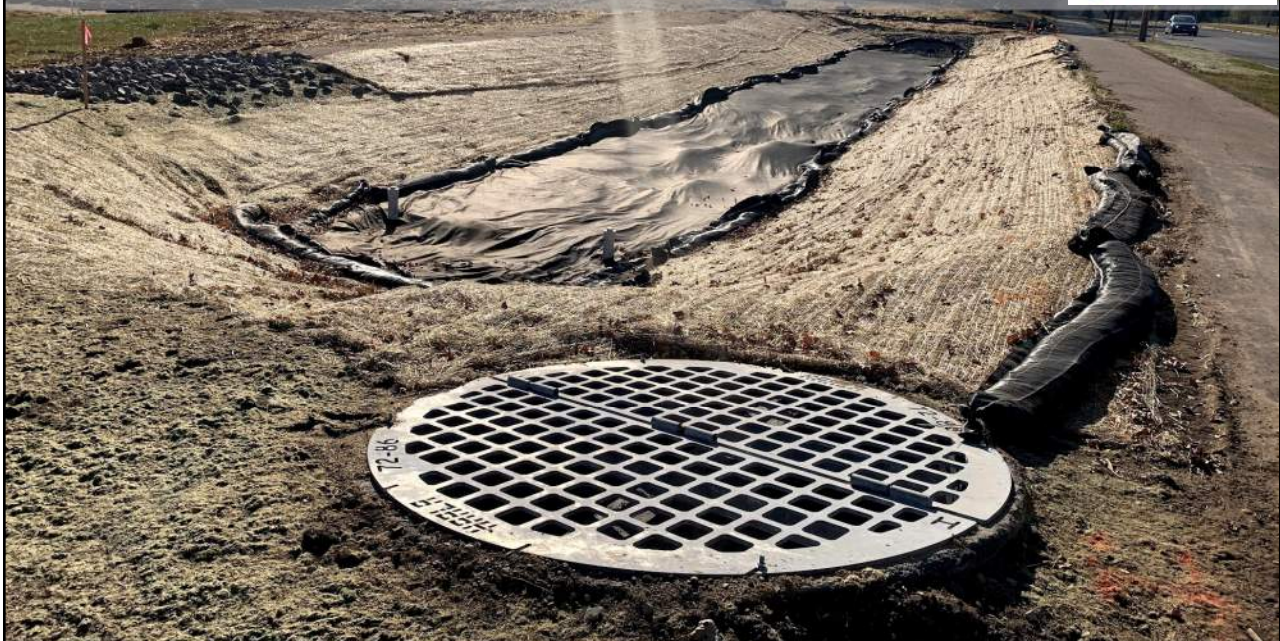
Basin Construction: Protecting Filter Media
