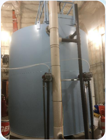
Solids Contact Clarifier
