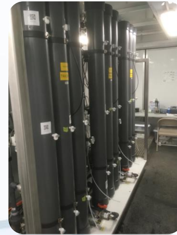
Disinfection Contactors (3 Trains)
