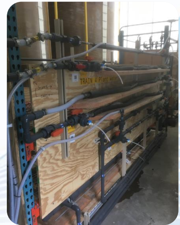
Pipe Loops (4 Trains x 2 Loops each)
