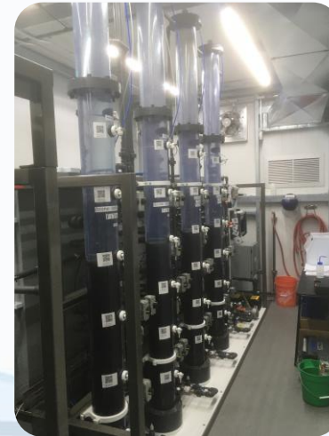
BAC Filters (4 trains x 2 each)
